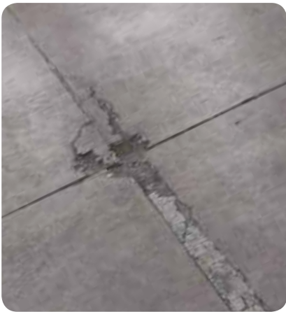
Spalling Joints
