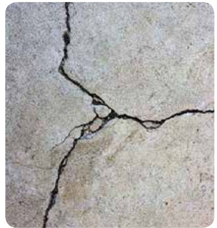
Wide Cracking
