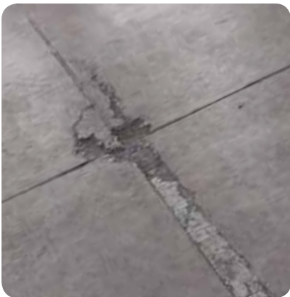
Spalling Joints
